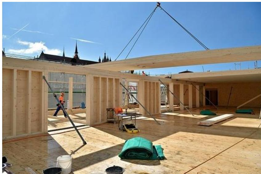
**Slika 2.** Modularni sistem drvene konstrukcije (<https://www.mdpi.com/2411-9660/2/3/30>)
